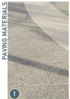
EXPOSED AGGREGATE AND BROOM FINISH CONCRETE
